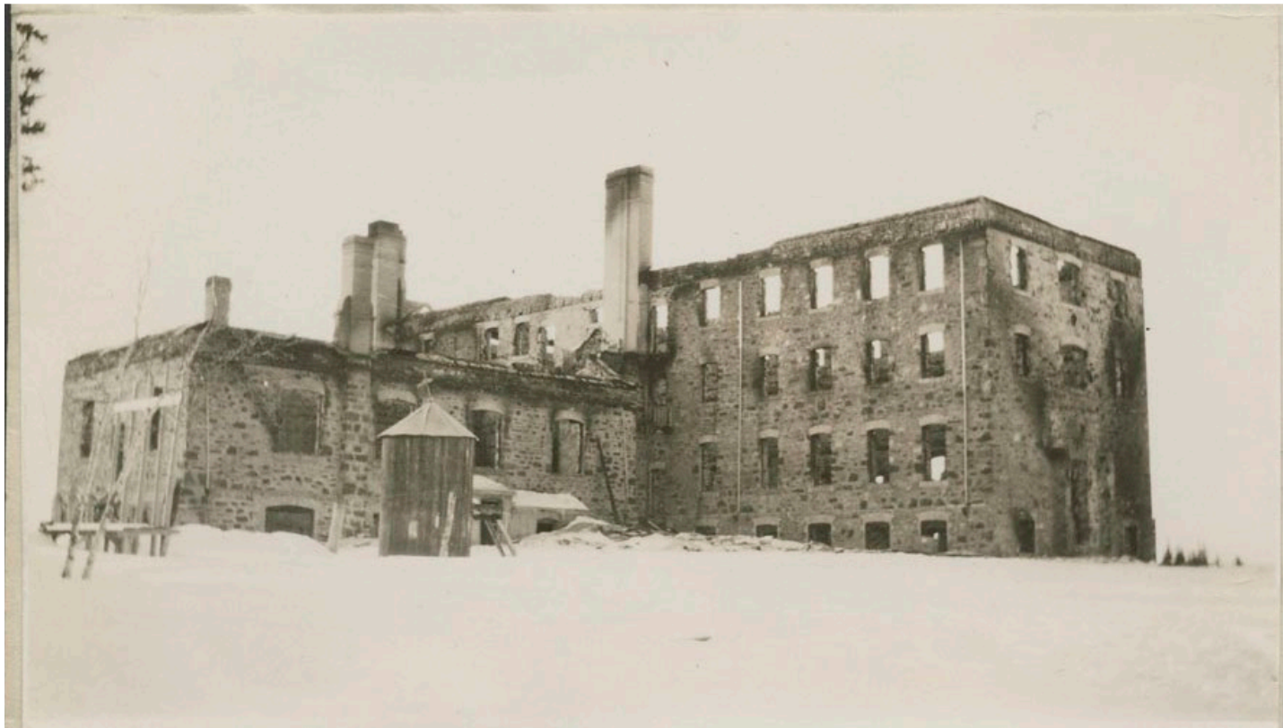
Cross Lake Indian Residential School burned stone building, Cross Lake, Manitoba, March 3–4, 1930. Photo courtesy of Library and Archives Canada.
